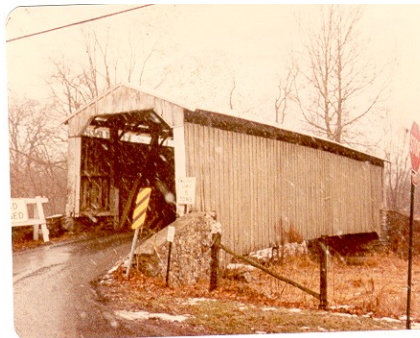
Bridge prior to 2002 arson fire
